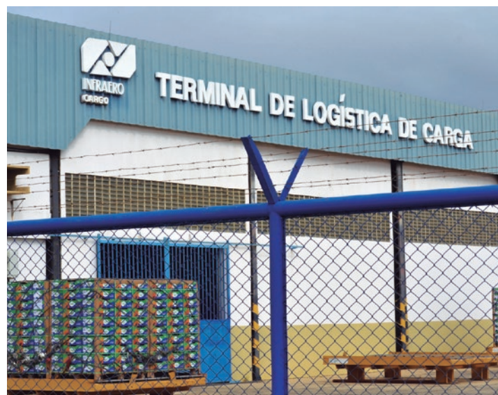
Freight Logistics Terminal of Petrolina (PE)
